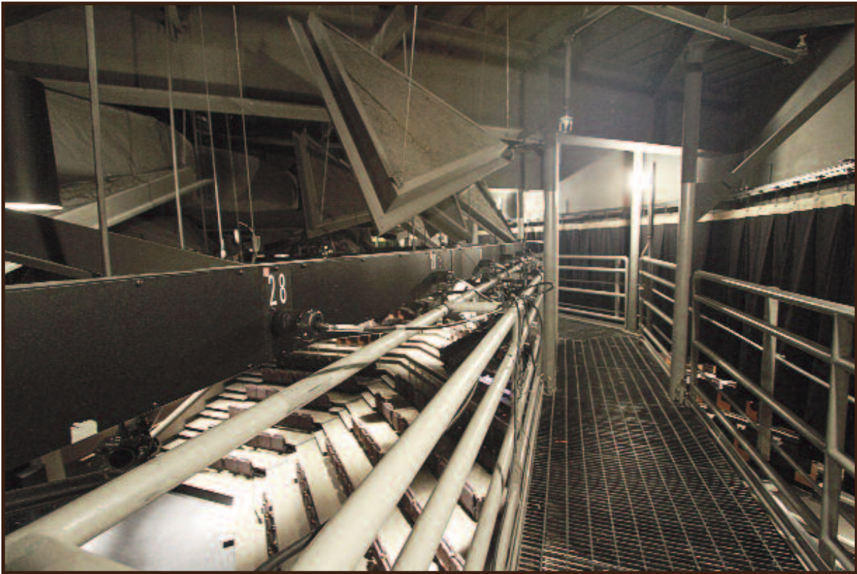
A 360° catwalk 21.5' above the floor rings the parterre and stage area.
