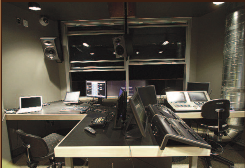
The control booth with an ETC Gio and fader wings on the right.
