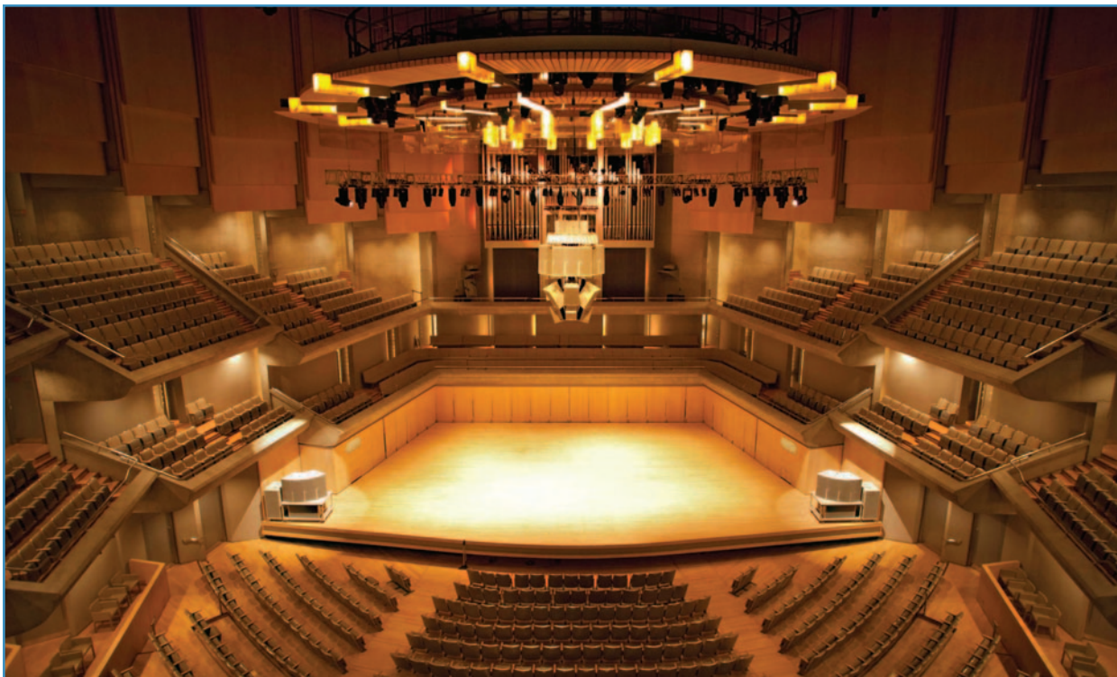
Stage of Roy Thomson Hall, showing new center cluster, acoustic reflector, deck-mounted L-R loudspeaker system, and staggered seating pods.
