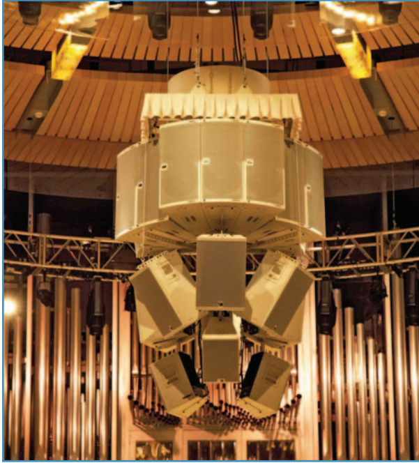
Center cluster redesigned to fit through the opening in the acoustic reflector above the stage.
