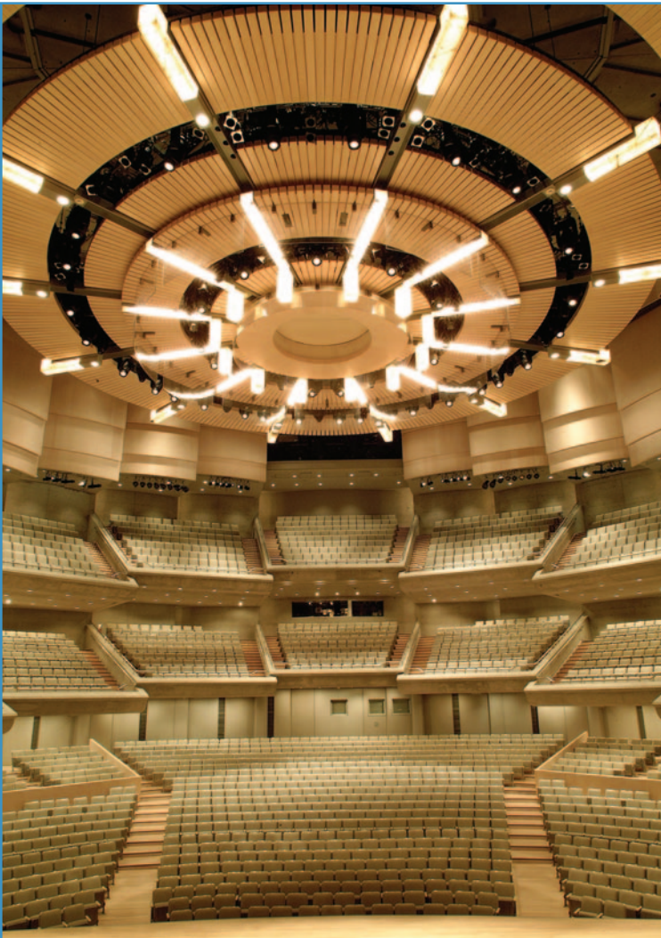
Wooden reflective canopy above the stage. Center cluster loudspeakers are retractable through a pair of doors in the center.
